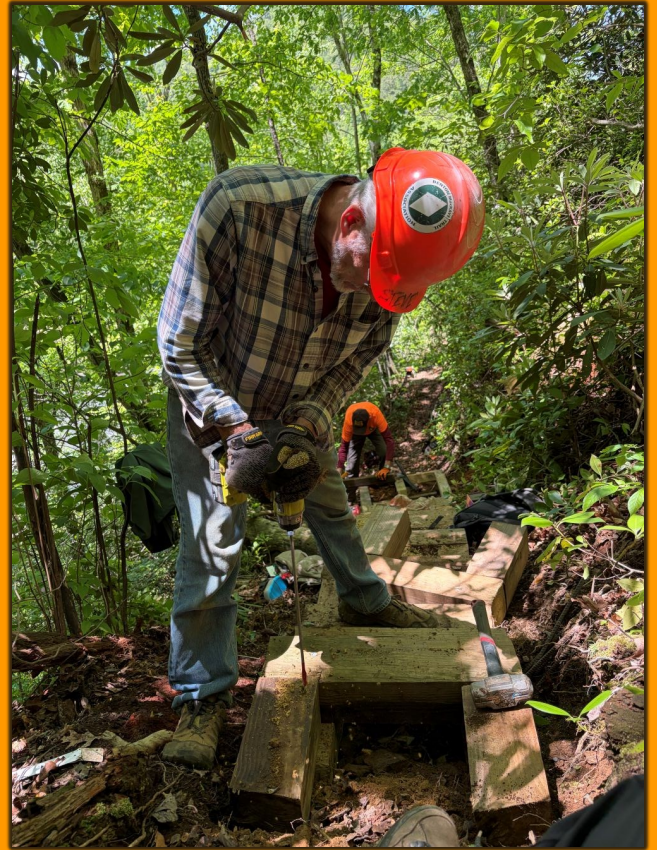
Steve Pruett drills steps into place.
